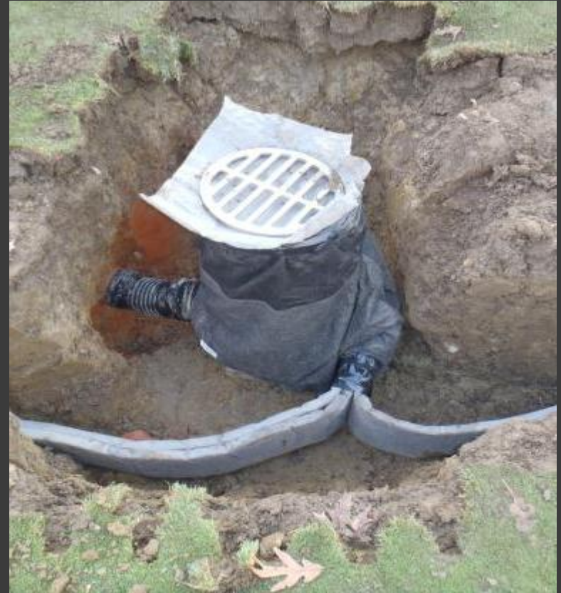
This allows seepage water to flow directly into the basin
