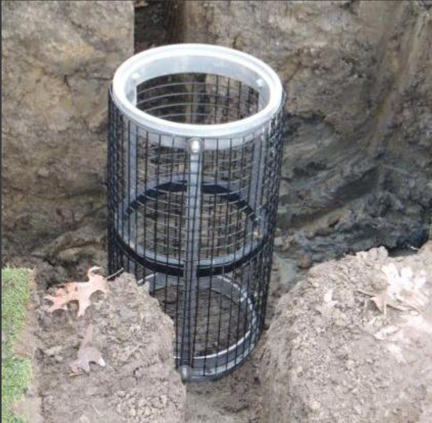
Geo Textile and sand surround the Perma Basin™
