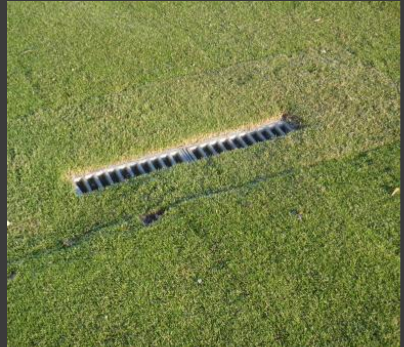
Channel Drain for concentrated flow
